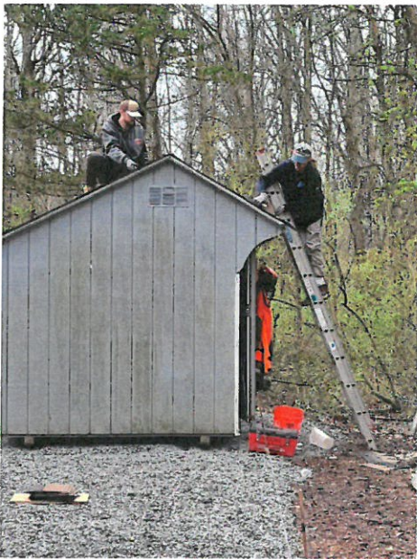
Habitat for Humanity roofers re-shingling gray shed.
