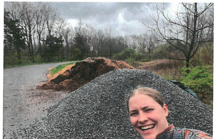
15 tons of gravel to be laid for shed foundations.
