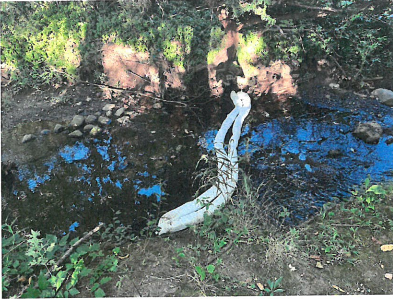
Figure 1: Absorbent sponges deployed along Loantaka Brook to collect the oil from the river
