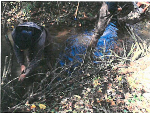
Instream woody debris being placed, cabled into the banks and additional woody material added to ensure sediment gets trapped at high and low water levels
