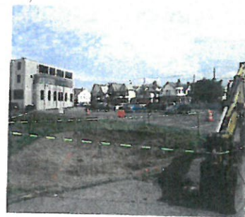
Above: Initial construction of previous school rain gardens, including depaving and excavation, has been done in the summer when schools were not in session. The drainage and permeable surfaces that will hold onto and slowly drain water into the groundwater are installed. The grade has been lowered and the sides sloped to encourage water to gather during active rainfalls. Left: Students at Great Swamp Wildlife Refuge learn about how creatures living in the stream can be indicators of good or poor water quality and what human actions can be taken to impact water quality. All photos by Hazel England
